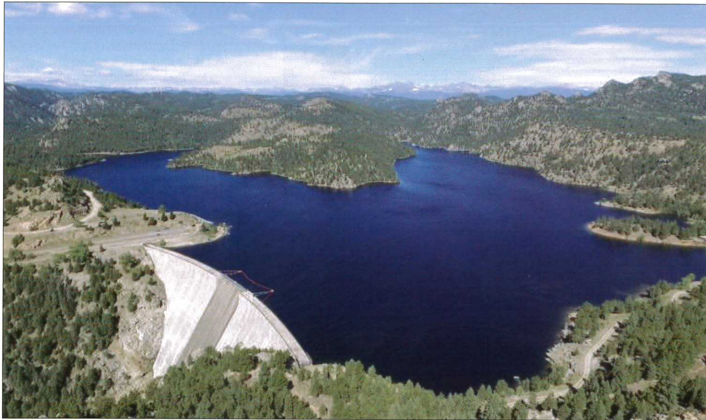
When completed, Gross Reservoir will be able to hold an additional 77,000 acre-feet of water—more than 25 billion gallons.
